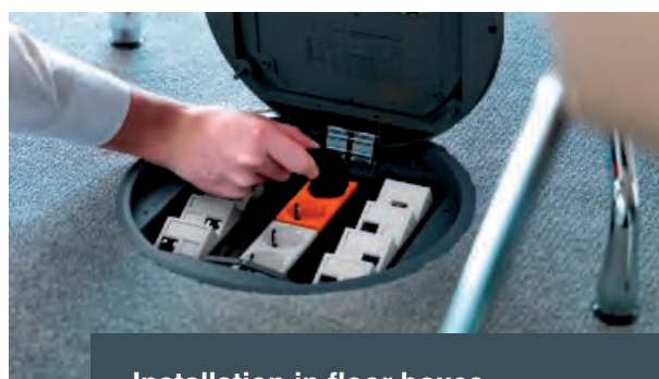
Installation in floor boxes
